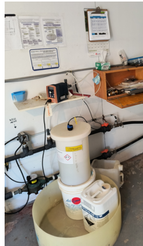
Figure 4 Chlorine Injection
