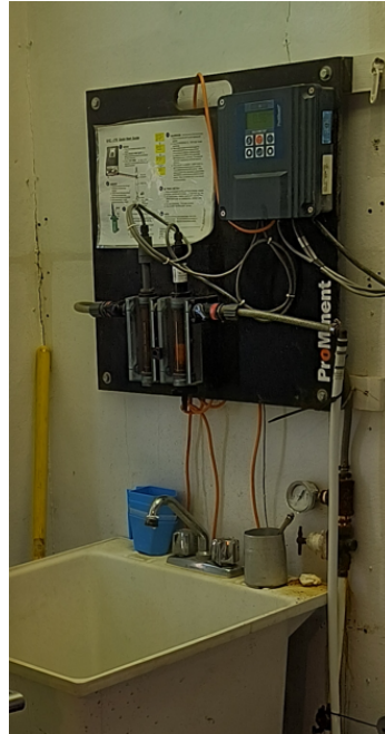
Figure 8 Chlorine Analyzer
