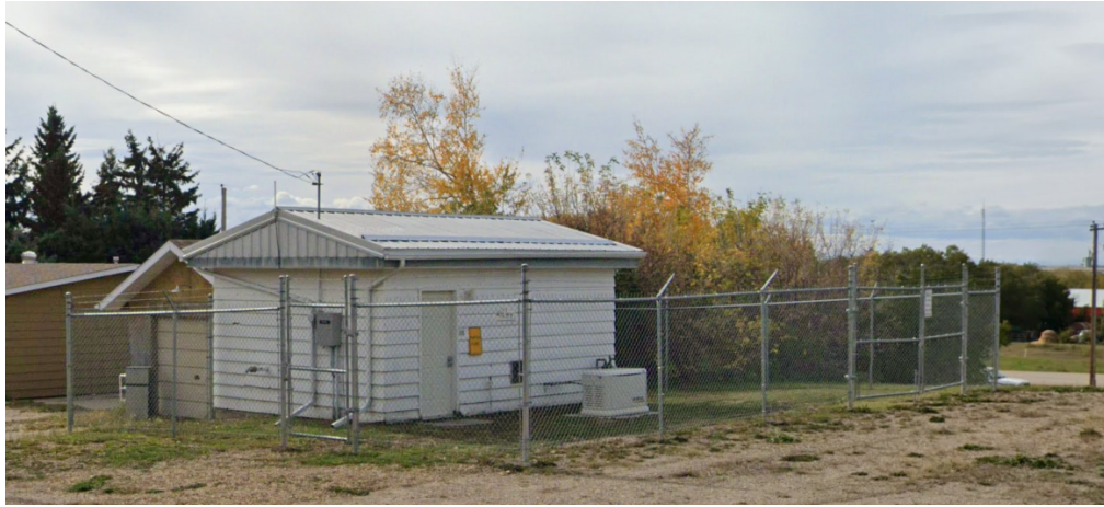
Figure 3 Water Treatment Building
