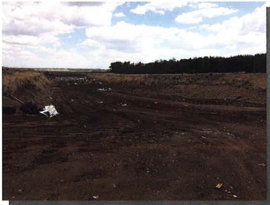
Photograph 6 – Looking East at Dry Disposal Cell 3
