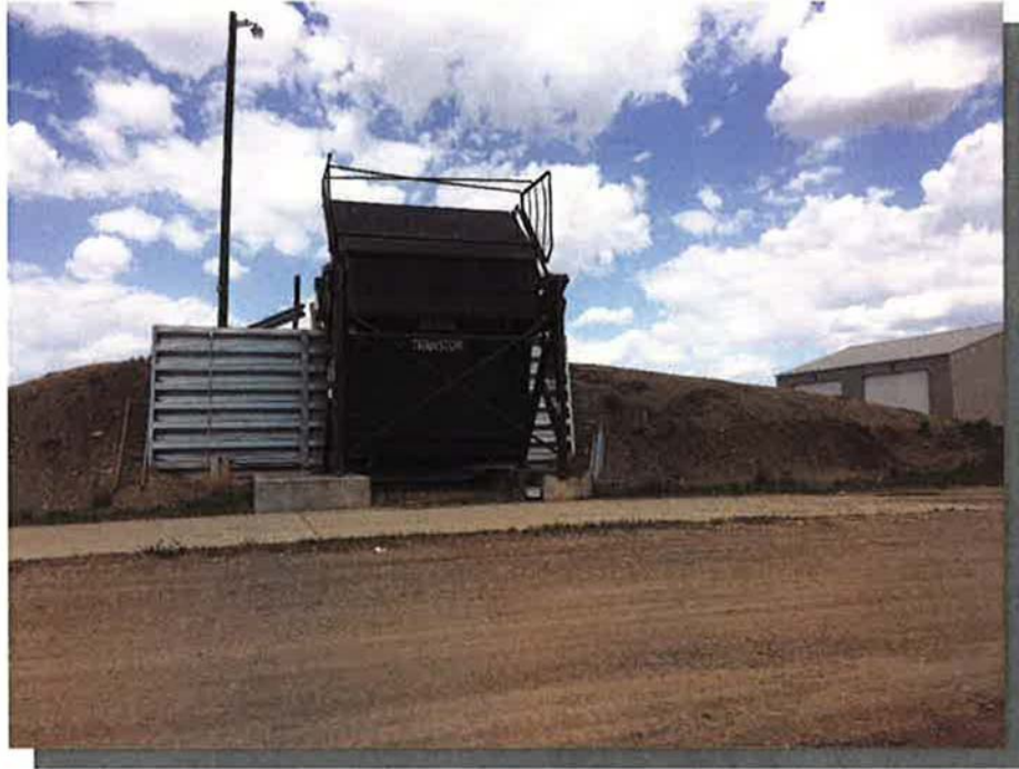
Photograph 5 – Looking North at the Compactor Pad
